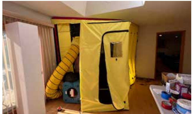
Sometimes you have to tape the containment to the wall.
