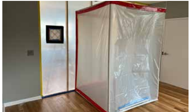
A properly sized containment will help maintain effective negative air.
