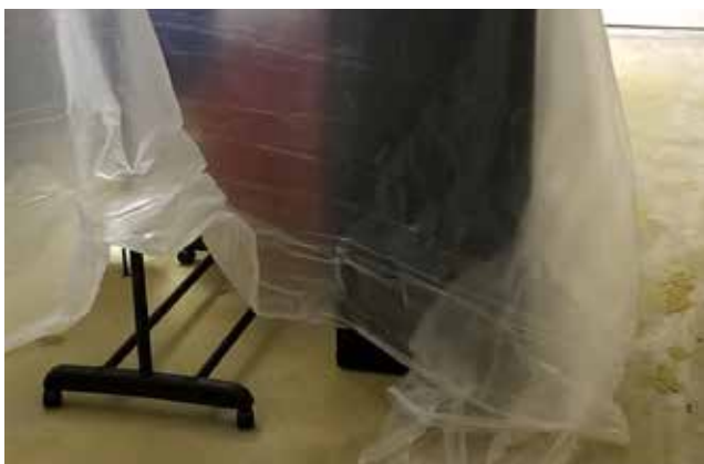
The image on the left shows an attempt to cover and protect some furnishing, and the one on the right shows how it failed because the loose-fitting plastic did nothing to stop dust buildup.
